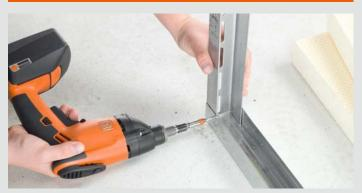
Hard torque-rate joints in drywall construction don't present a problem thanks to the acceleration switch and robust design, making the FEIN drywall screw guns ideal problem-solvers – in all areas.
