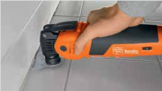
Removing elastic grout sealants.
