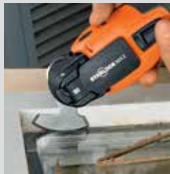
Cutting out putty-mounted insulation glass windows.
