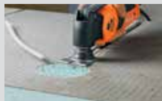
Preparing for electrical installation.
