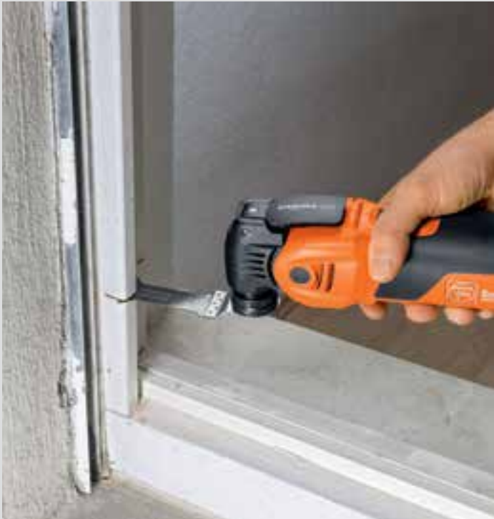
Cutting through window frames.
