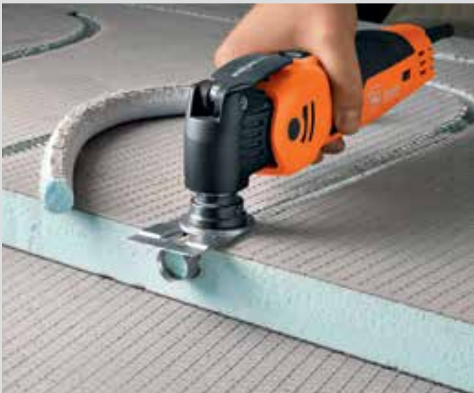
Cutting out channels for hot water underfloor heating.
