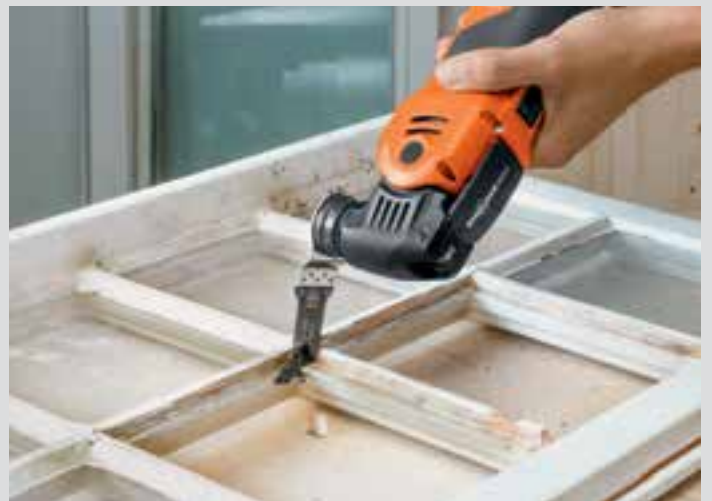
Restoring old windows.
