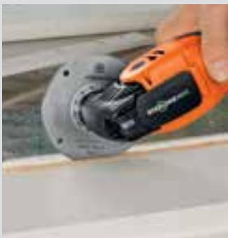
Cutting through nails on window bars.
