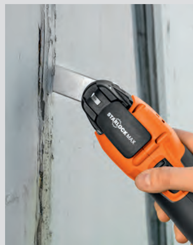
Removal of flexible joint sealants in above and below-ground construction.
