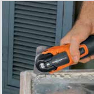
Oscillation motion eliminates risk of glass breakage.
