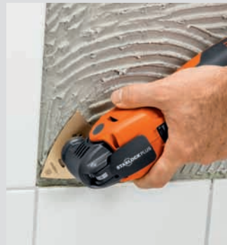
Remove tile adhesive with rasp.
