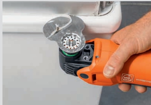
Remove connection joints.
