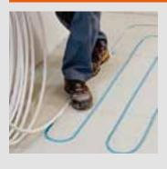
A 1/2 or 3/4 inch plastic water pipe is laid in the individually made cut-out (Ø approx. 25 mm).
