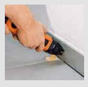
Sawing flush to pipes
