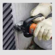
With the diamond cleaning blade, the extraction device can be used to roughen mortar flanks as well as remove the sealant material.
