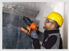
Chiselling Remove excess concrete.
