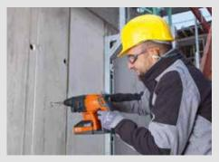
Hammer drilling Hammer drill up to 20mm in concrete.
