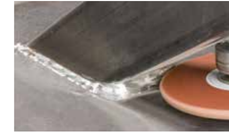
Grind the welded seams in hard-to-access constructions
