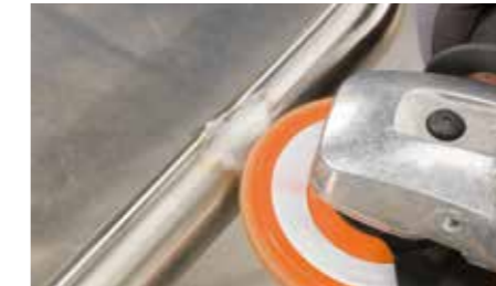
Removal of the welded seam without damaging the adjacent surface
