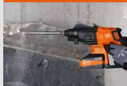
Remove excess concrete.
