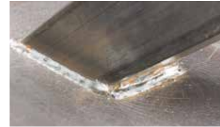
Unmachined welded seams with tarnishing in metal constructions
