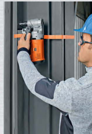
Even vertically and overhead
