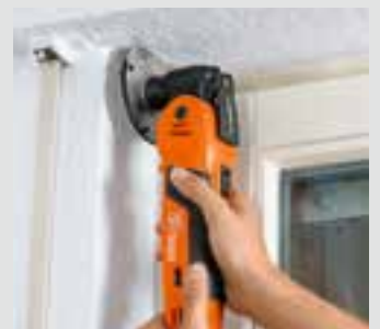
Cutting open covers on roller shutter cases.
