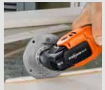
Cutting through nails on window bars.
