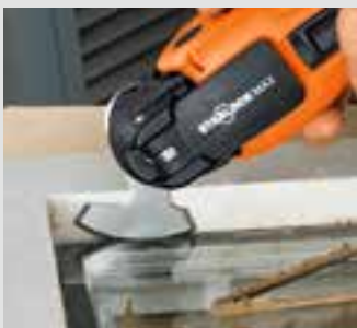
Cutting out putty-mounted insulation glass windows.
