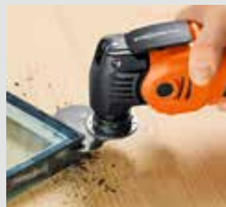
Separating insulating glass.
