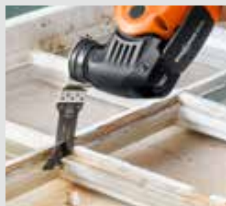
Restoring old windows.
