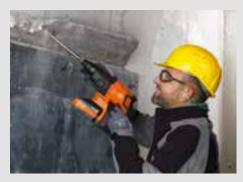
Chiselling Remove excess concrete.
