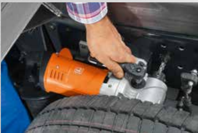
Optimum view of drilling point
