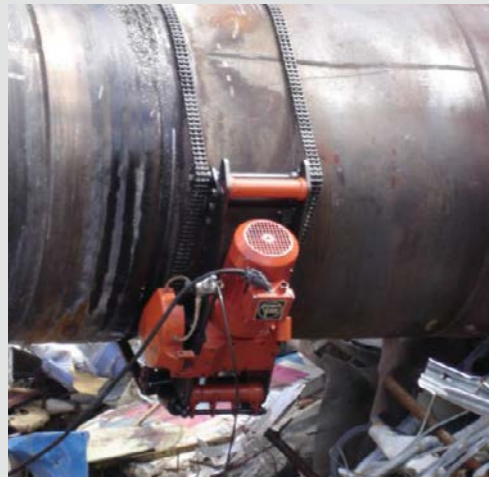
In tank construction.
